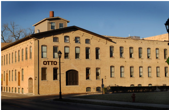
The OTTO facility in Carpentersville, IL
